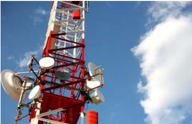
GENCO ATC uses Warehouse Management to support on-the-fly operational changes in the dynamic High Tech/Wireless Industry.
